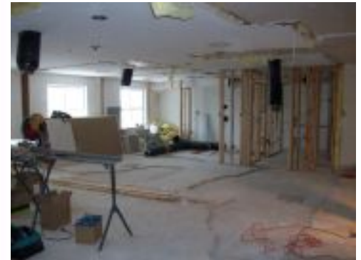
Construction crews continue to work on the new Manor Activity Center.
